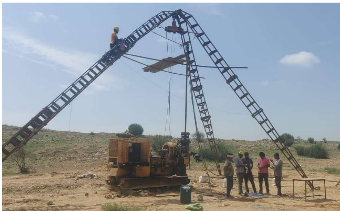
Photo-12.2 Photograph of RD-100 Drill Rig
