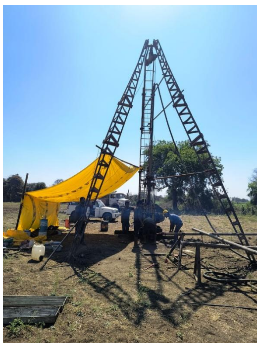
Photo 08: Photograph showing conventional drill rig (RD- 60) MEC- 347 at Borehole no. MHG-01.
