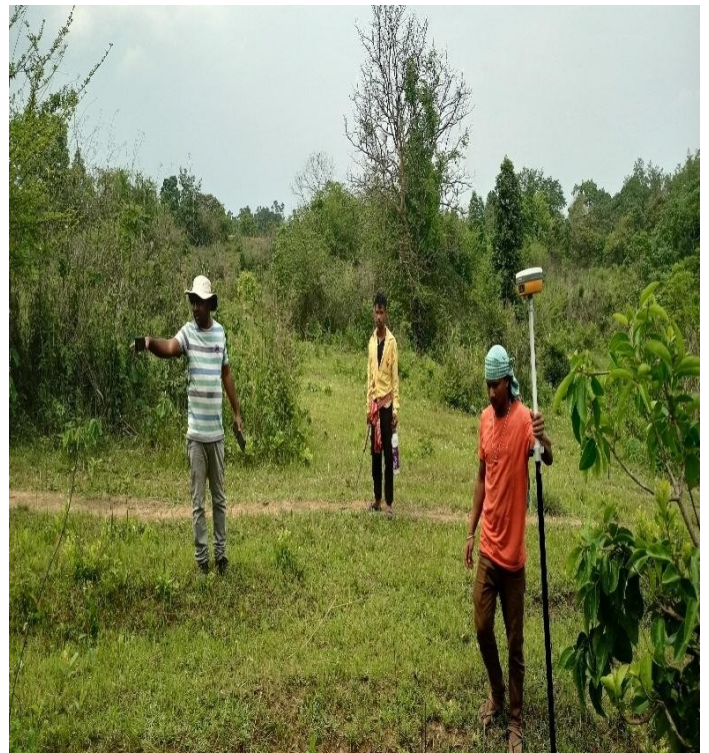
Fig.5.2: Topographical survey done by DGPS
