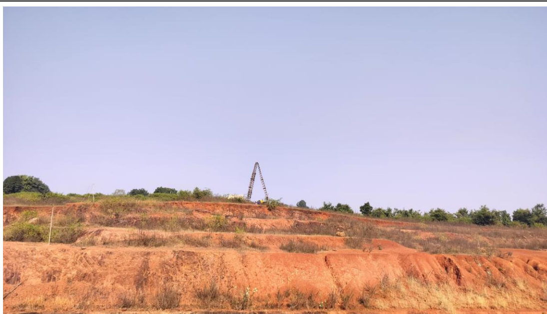
Panoramic view of MECL drilling rig on Lateritic benches at borehole location MBM-4
