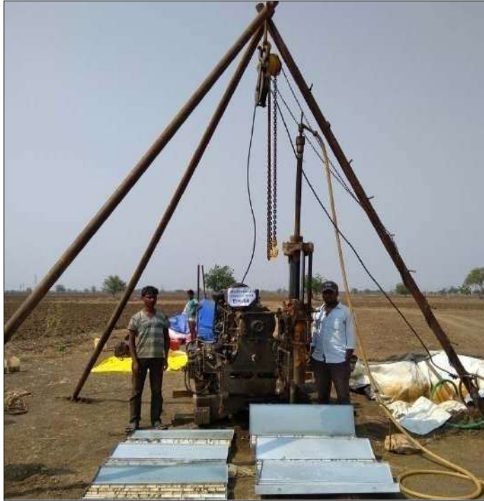
Figure 3.1 Core drilling in Madinapadu limestone block
