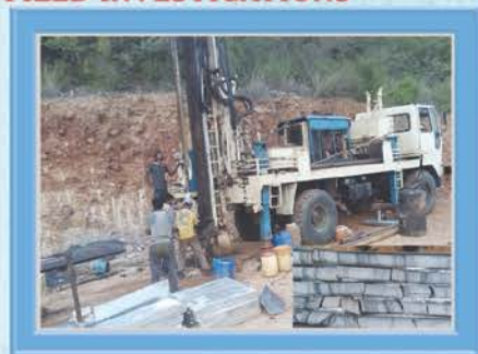
Core drilling in Mangampeta
