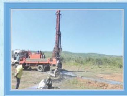
Non-core drilling in Kadapa district
