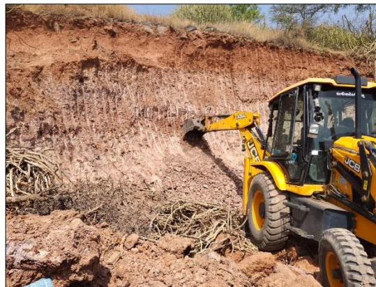
Photo No – 4: 2.39 km east of Lakhond. The uppermost part is composed of hard, compact ferruginous sandstone, which is underlain by laterite and bauxitic clay at the bottom.
